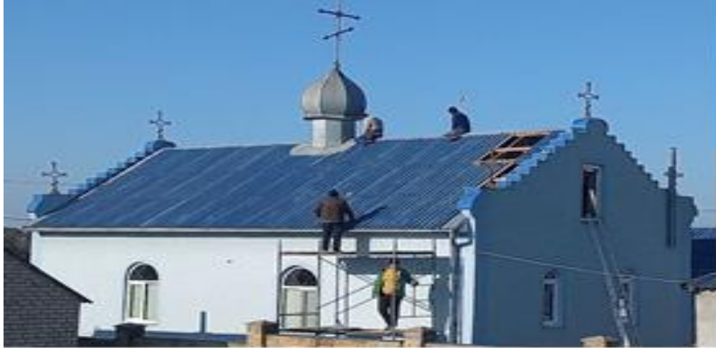
Repairing the Orthodox Church
