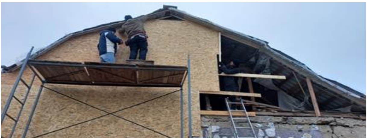
Emergency repairs to badly damaged adjacent buildings
