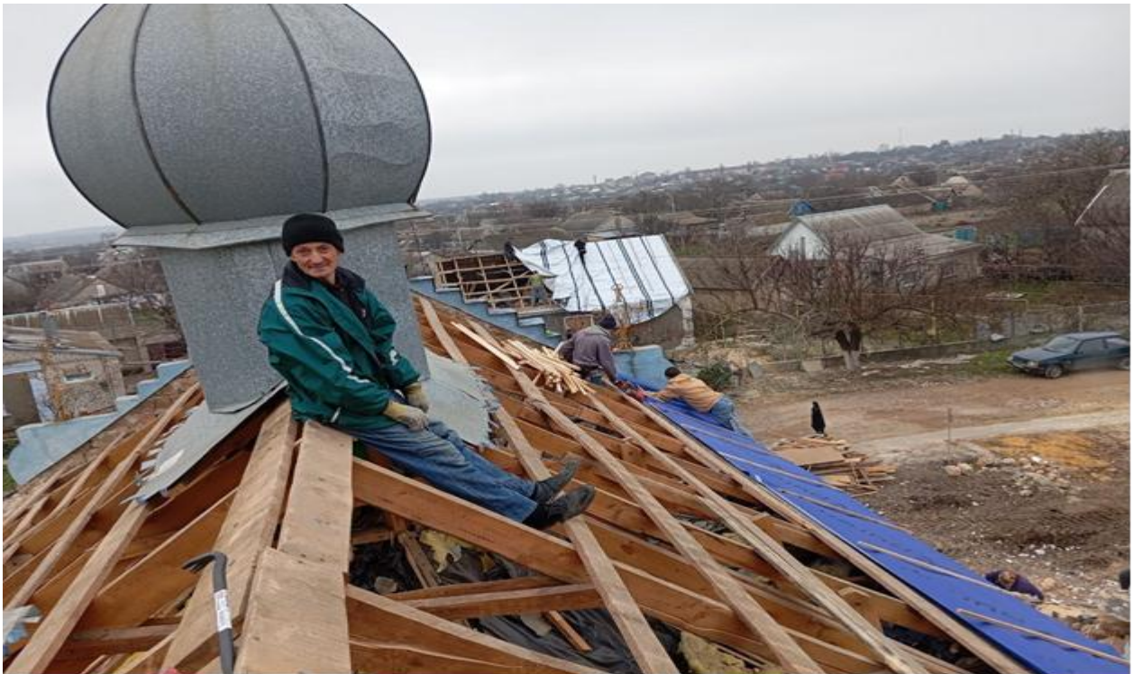
Orthodox Church – roof repair team at work
